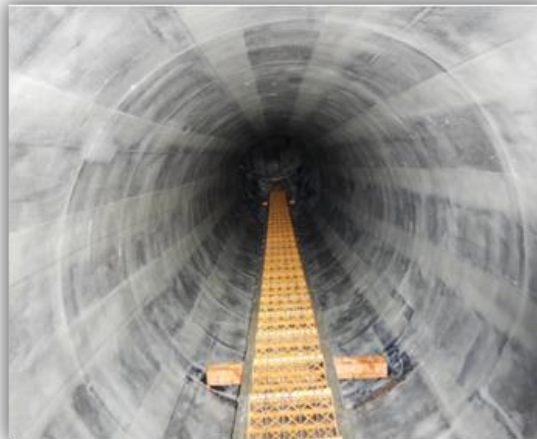
Watertightness layer
