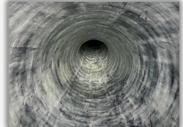
Topcoat and curing
