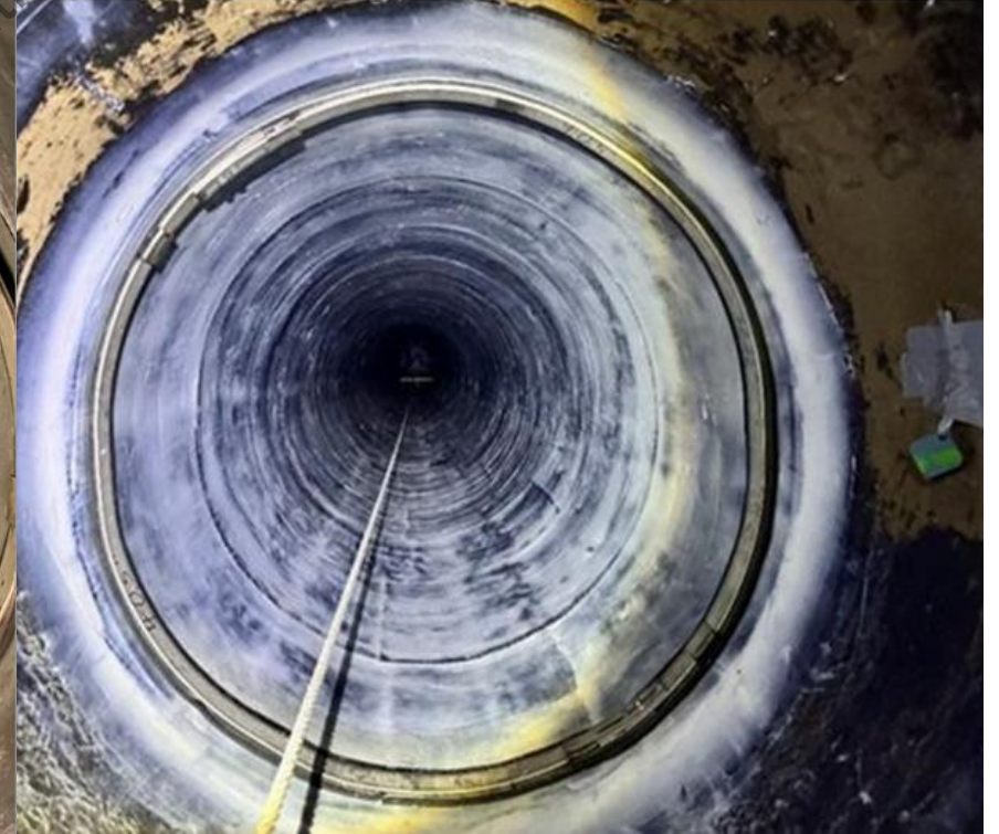
Watertightness layer & final topcoat & expansion ring termination
