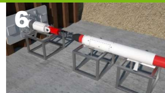
3 Handling & coupling of temporary steel jacking pipes
