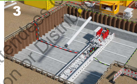
3 Handling & coupling of temporary steel jacking pipes
