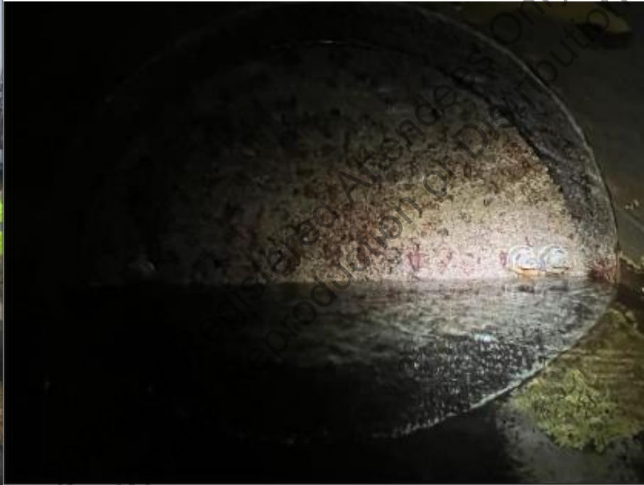
High water level
