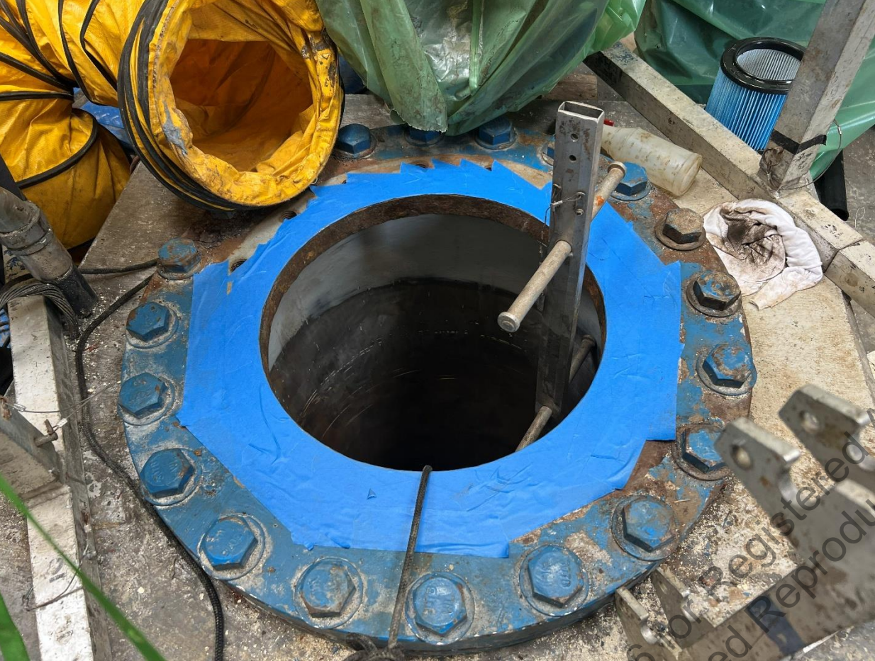
Hand Coated 1 st Ft. (Welds)
