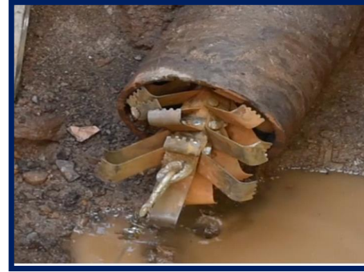
PIPE CLEANING, PREPARATION AND DRYING WITH TOMAHAWK AIR-DRIVEN STONE PROCESS.
