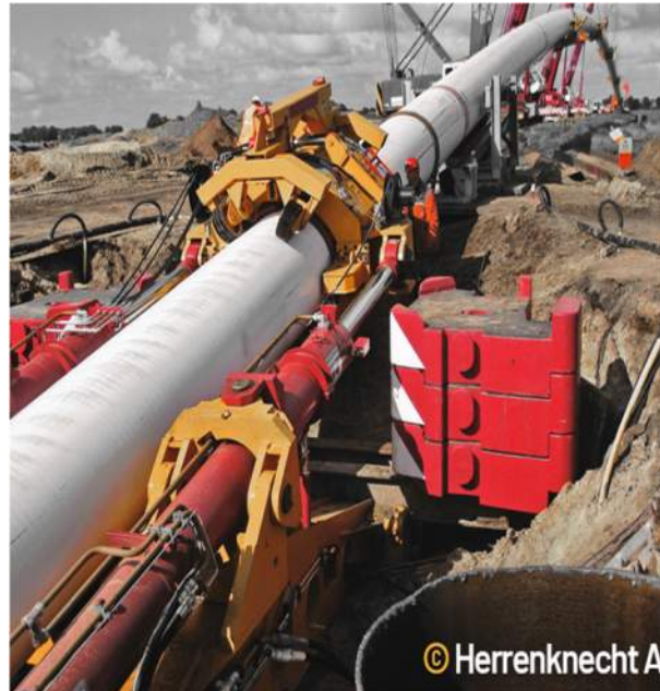
Direct Steerable Pipe Thrusting
