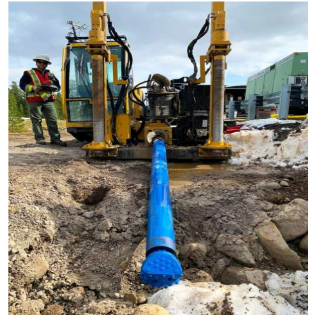
Horizontal Directional Drilling
