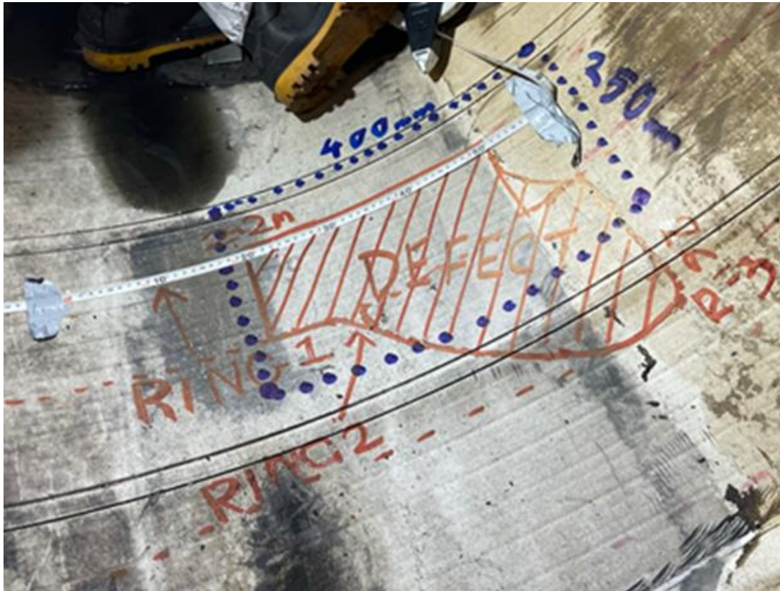
Mapping flaw – pipe invert
