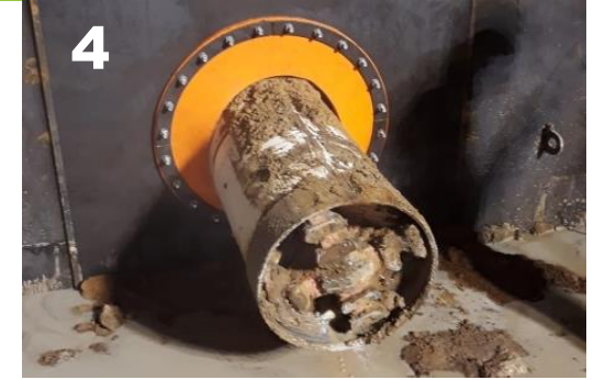
4 Precise breakthrough at target point
