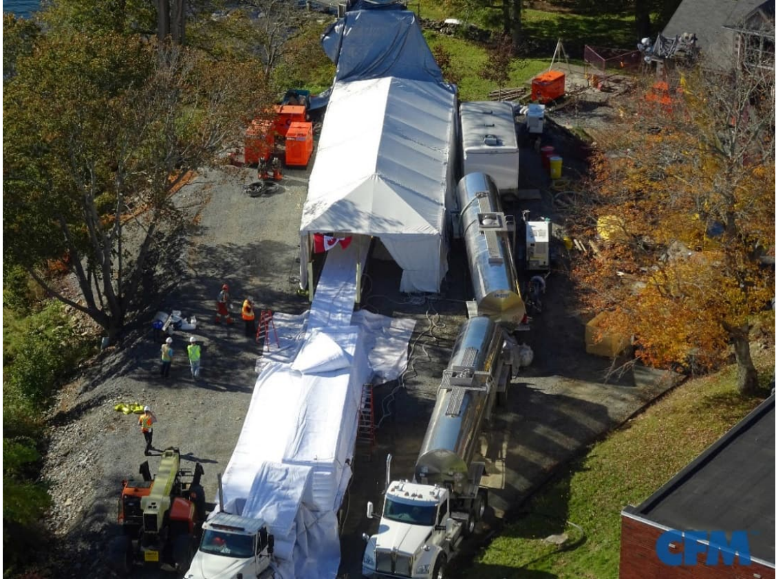
0% On-Site/Over the Hole Wet-Out
