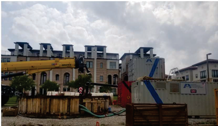
MTBM Control Cabin and Power/Hydraulic Containers
