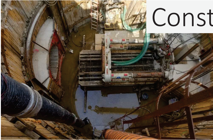
Jacking Frame (Without Microtunnel Boring Machine)
