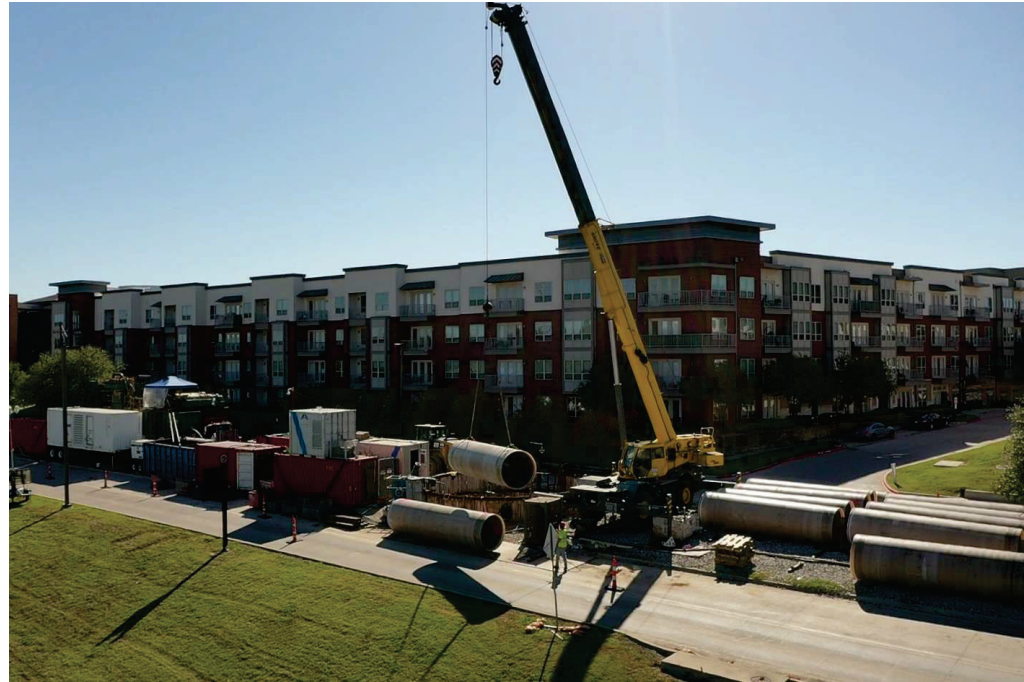
Lowering 60" FRP into Jacking Shaft
