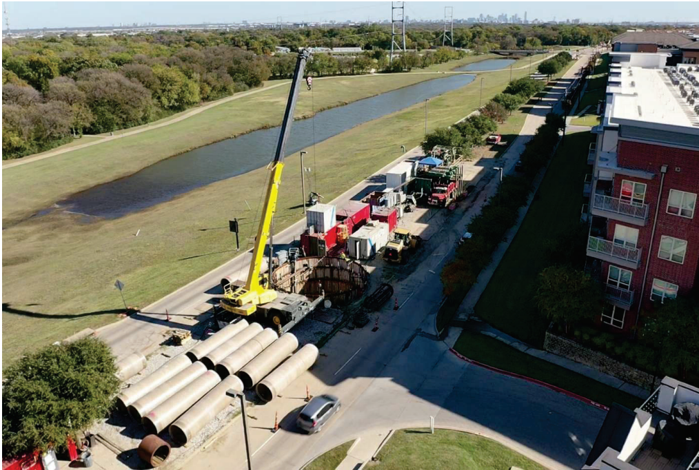
Staging Area for Microtunnel Drive
