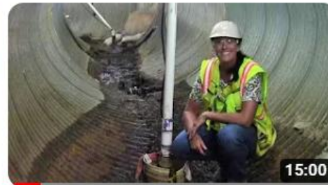
CCCP to the Rescue! 84-inch Storm Drain Rehabilitation, Kaua'i
