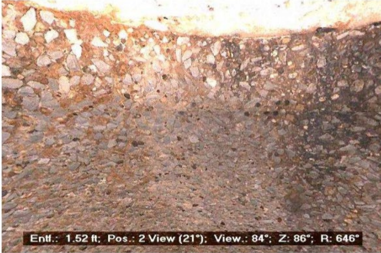
Surface Aggregate Visible – MACP Score 3
