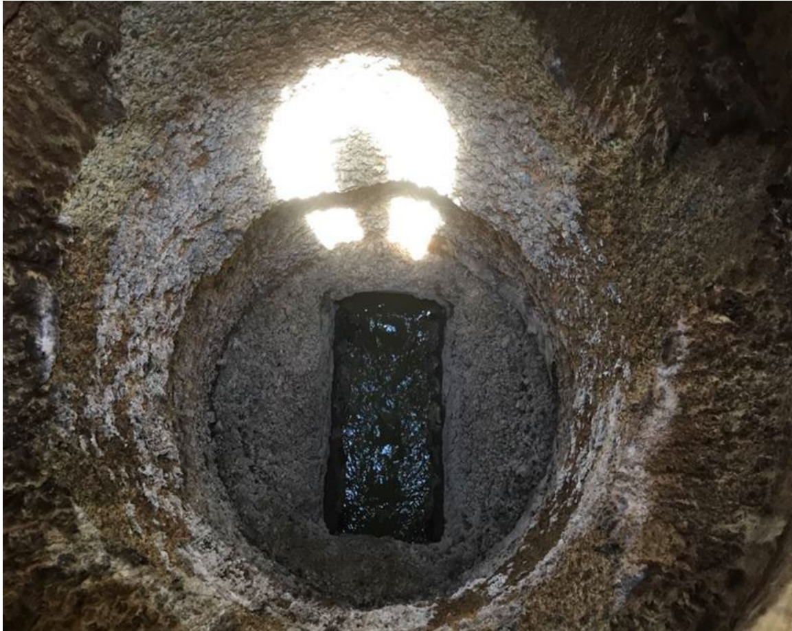
Surface Aggregate Projecting – MACP Score 3
