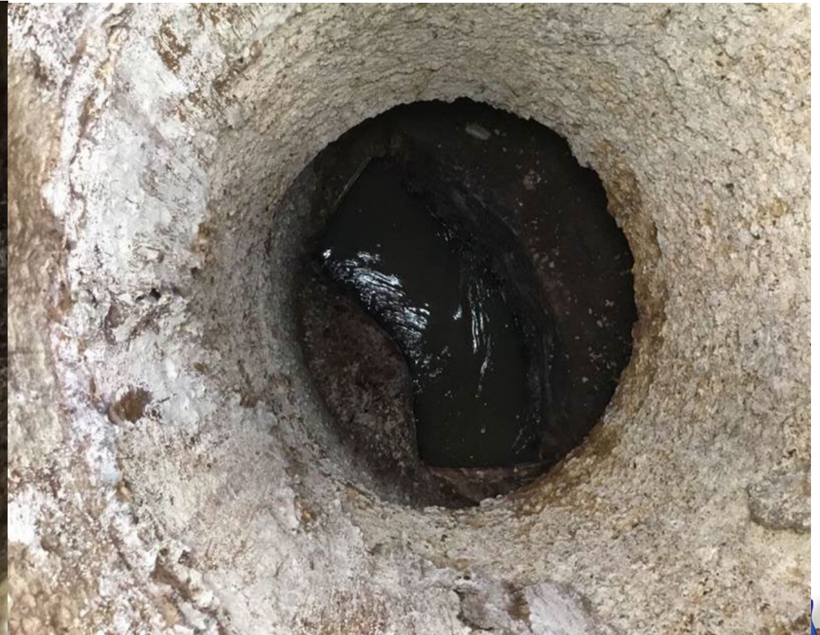
Surface Aggregate Projecting – MACP Score 3
