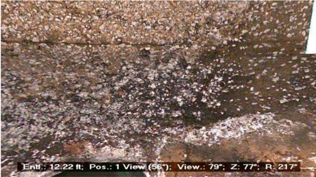
Surface Aggregate Missing – MACP Score 4
