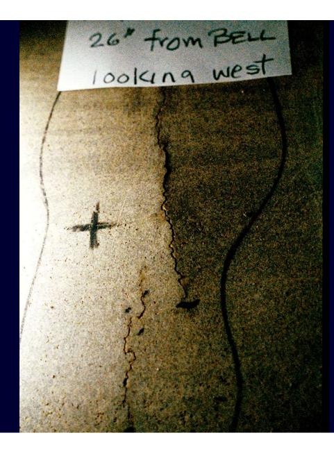
Invert crack about same distance from bell end of pipe.
