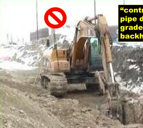
"contractor pushing pipe down to grade with backhoe bucket"
