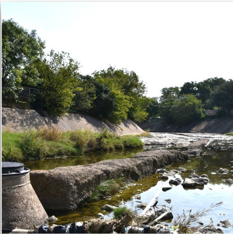
Concrete cap on existing line inside creek and channel
