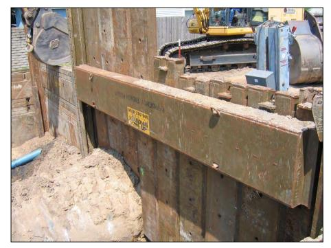
Generation 1.0: Utilize 2' wide steel panels, pinned in frame
