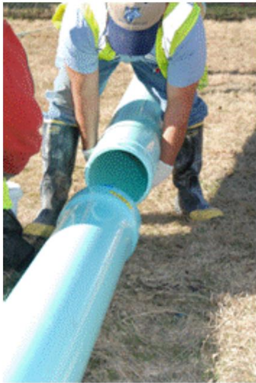
Clean, lubricate & assemble joint
