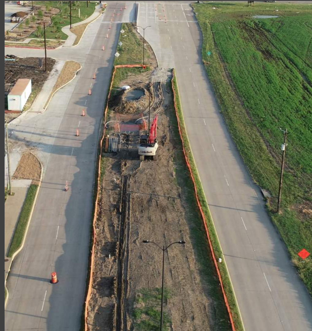
Drill Rig Staging Exit Pit
