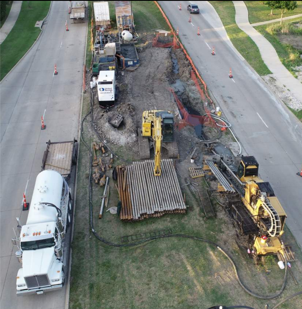
Drill Rig Staging Entry Pit
