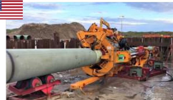
# 26 Sur de Texas Tuxpan Pipeline, Texas, 42", 4,900ft gas pipeline landfall (2017)
