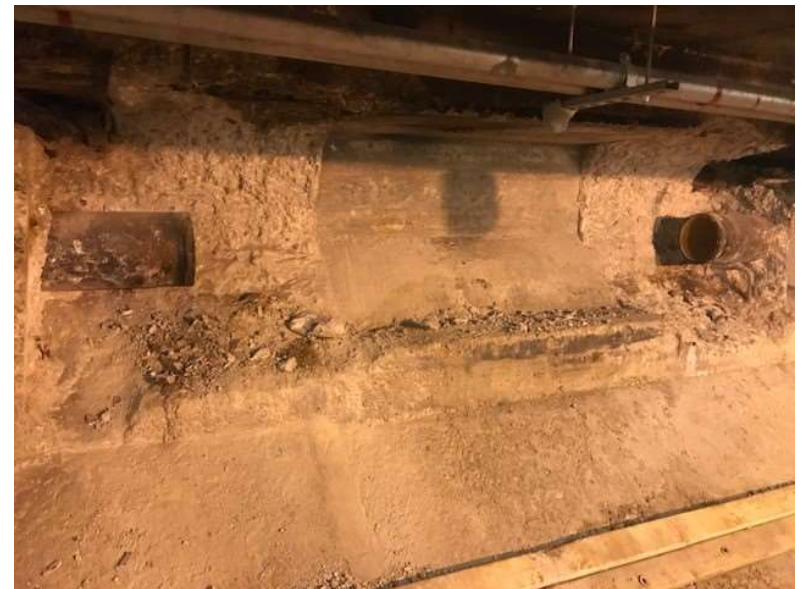
Example of concrete removal
