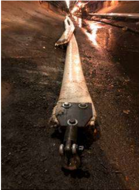
Pull head on staged liner
