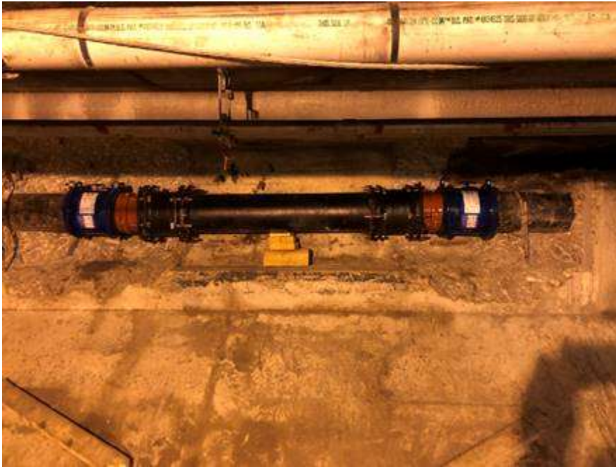
Fully completed installation with tie-ins
