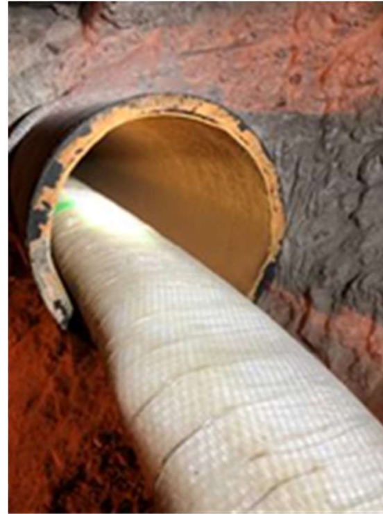
Liner – pulled-in, uninflated
