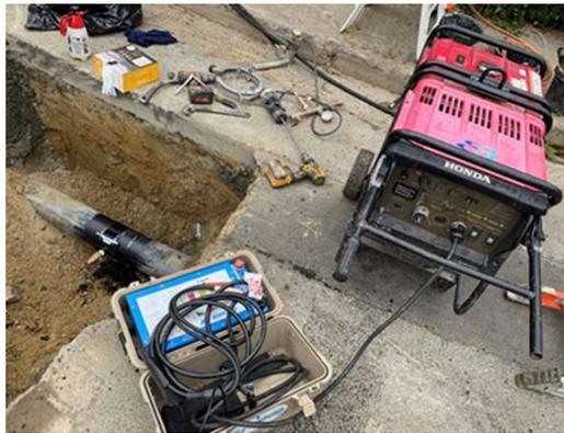
Typical Tooling Required For EF Saddle Installation
