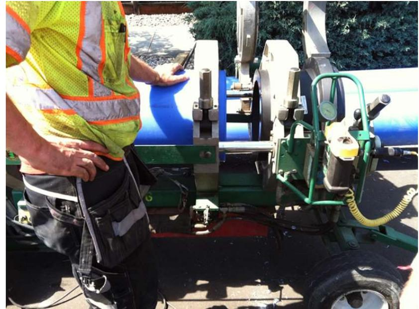
14" Butt Fusion/MJ Joint Adapter Fitting
