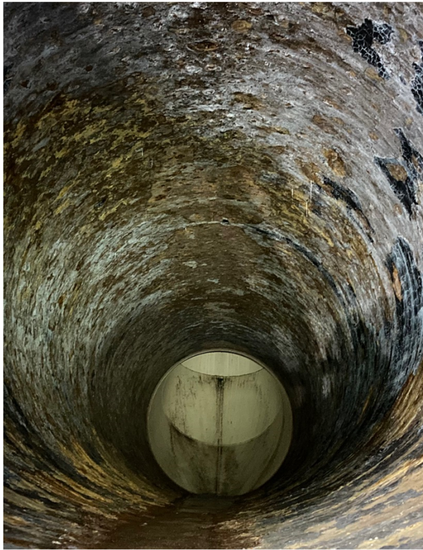
NESPS 72-in dia. Pump Discharge Pipe Corrosion
