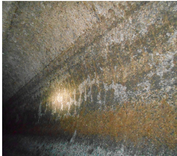
17.5 ft. dia. NI-EA Sewer Concrete Deterioration d/s of NESPS
