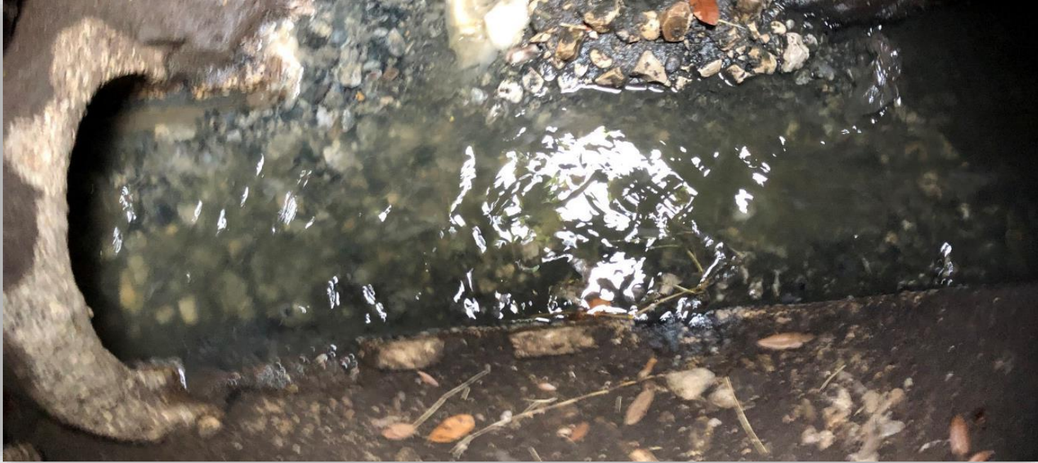
Gravel and Rocks Observed in Manhole Channel Cleaning pushed debris to next segment
