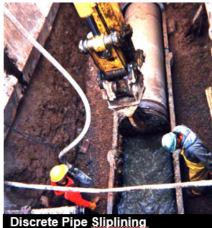
Discrete Pipe Sliplining
