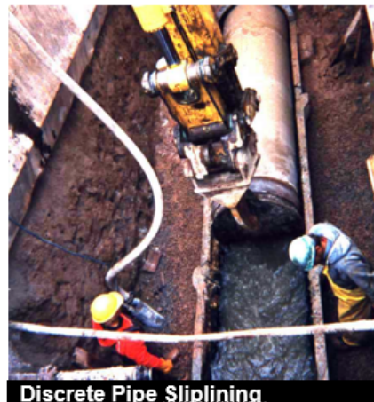
Discrete Pipe Sliplining
