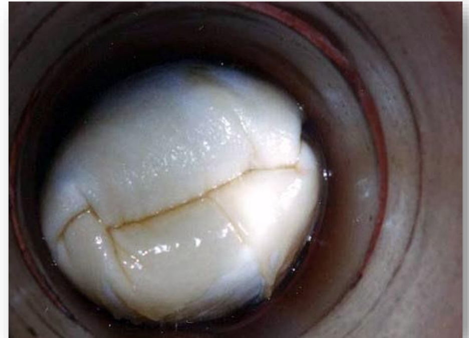
CURED-IN-PLACE-PIPE
