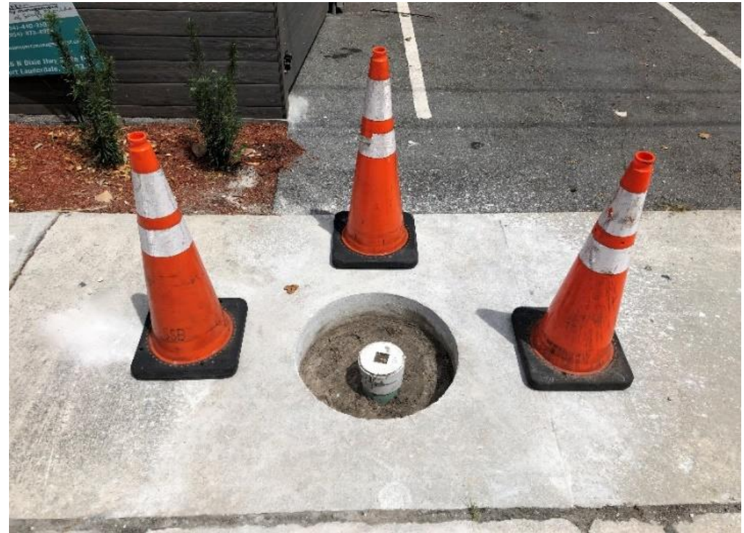
ASTM F3097 Minimally Invasive Cleanout In Sidewalk
