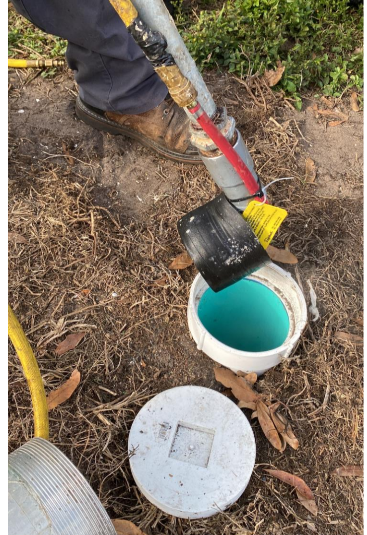
Figure 4 Cleanout Pump-through Plug
