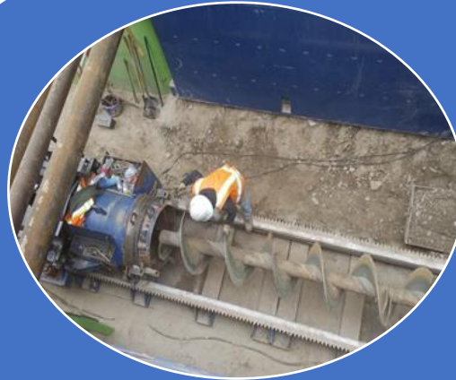
HORIZONTAL AUGER BORING
