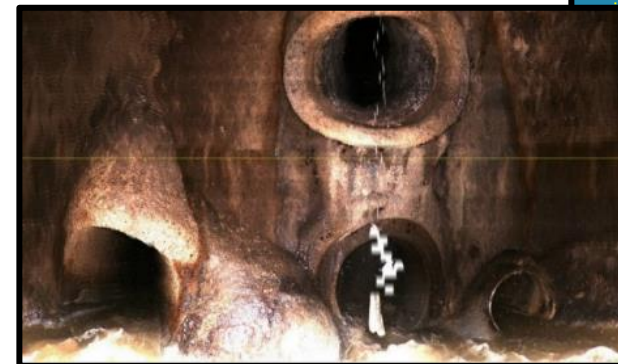
Digital Manhole Inspections
