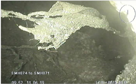
Collapsed pipe
