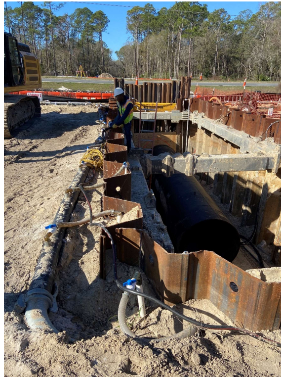
Well Point System around Launch Shaft
