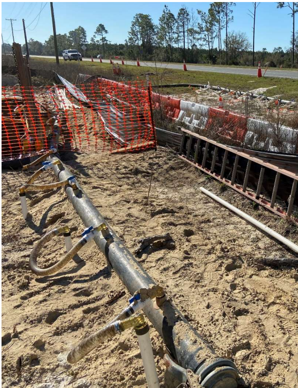
Well Point System around Launch Shaft
