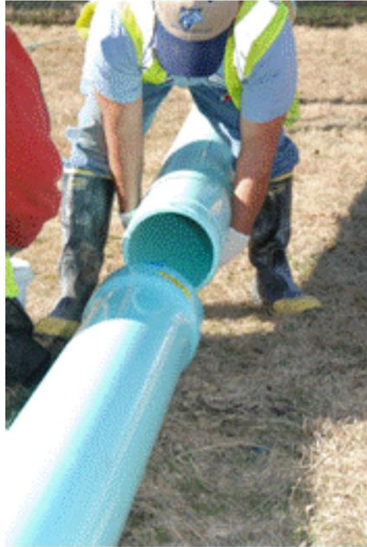
Clean, lubricate & assemble joint
