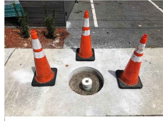
Minimally Invasive Cored Sidewalk
