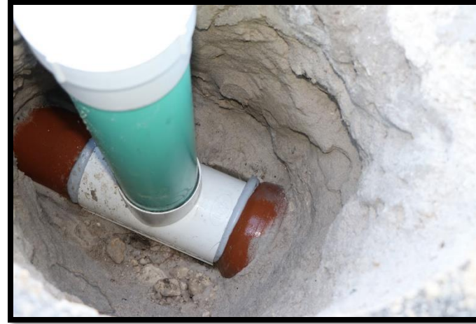
Vacuum Excavated Cleanout
