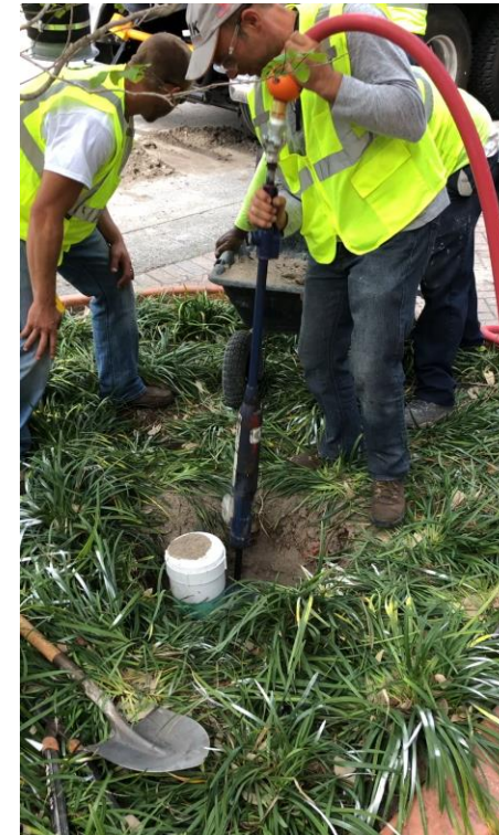
Compacting Trench Fill
