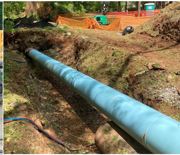
Conventional Sliplining HDPE & Fusible PVC
