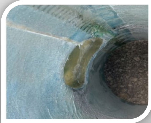
InnerCure system after lining of CIPP mainline liner (post reinstatement)
