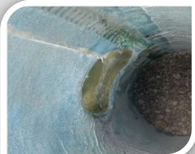
InnerCure system after lining of CIPP mainline liner (post reinstatement)
