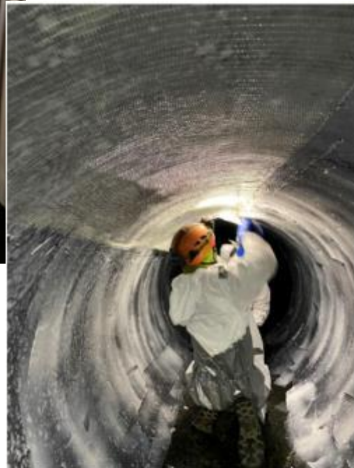
Figure 4 - Installing EG50 Longitudinal on S&P Segment
