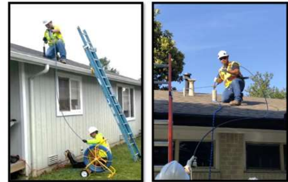
Figure 20: Roof vent inspection with manual push camera. Fall protection must be used according to safety regulations.
