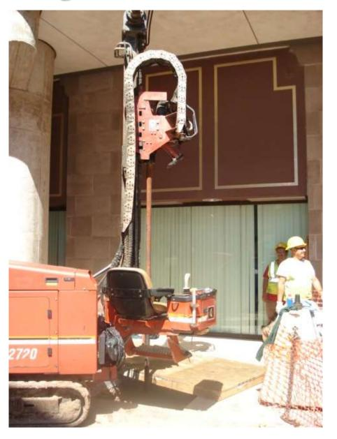
This machine can make deep large diameter saddle taps
