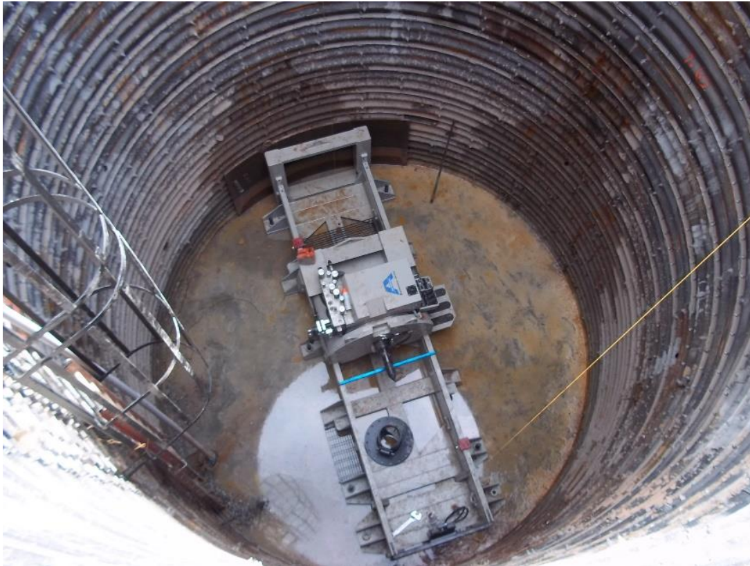
Akkerman Model 4800 installed in a jacking pit
