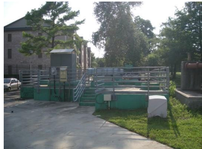
Dairy Ashford Lift Station Site
