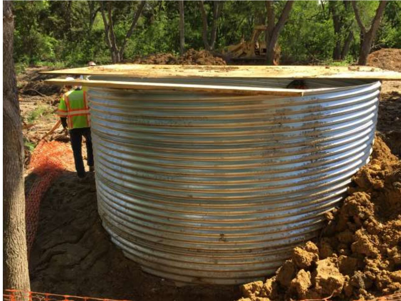
Tinhorn Manhole Installed at Both Ends of Bypass
