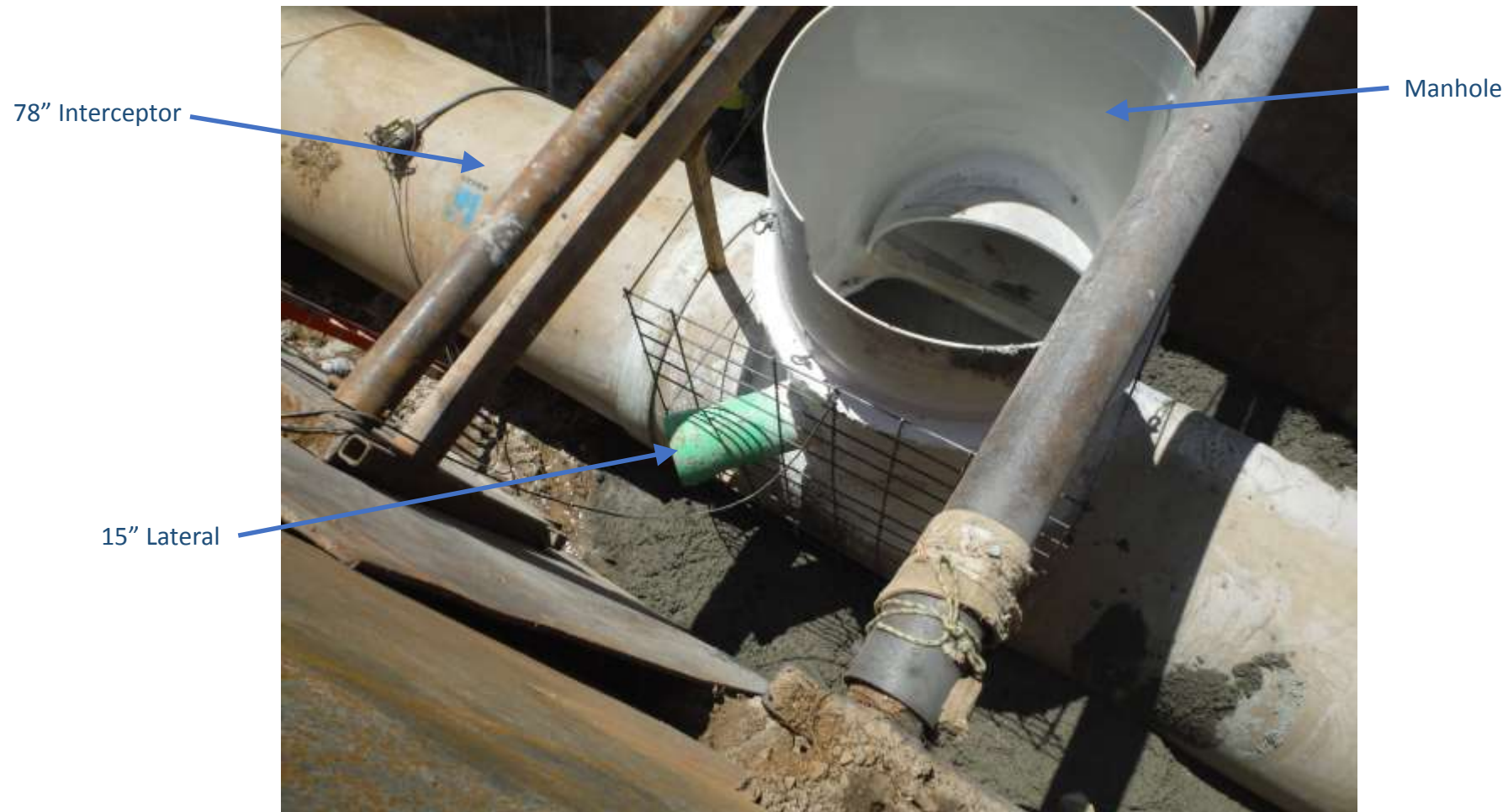
View of 78" WWMH From Above
