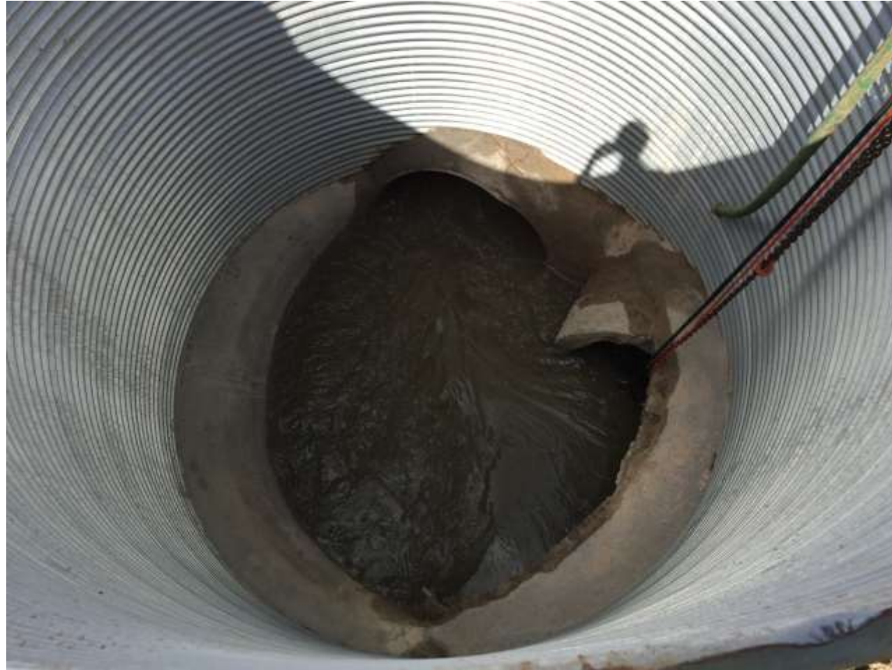
Upstream View of the Bypass Installed at Crossland Blvd.
