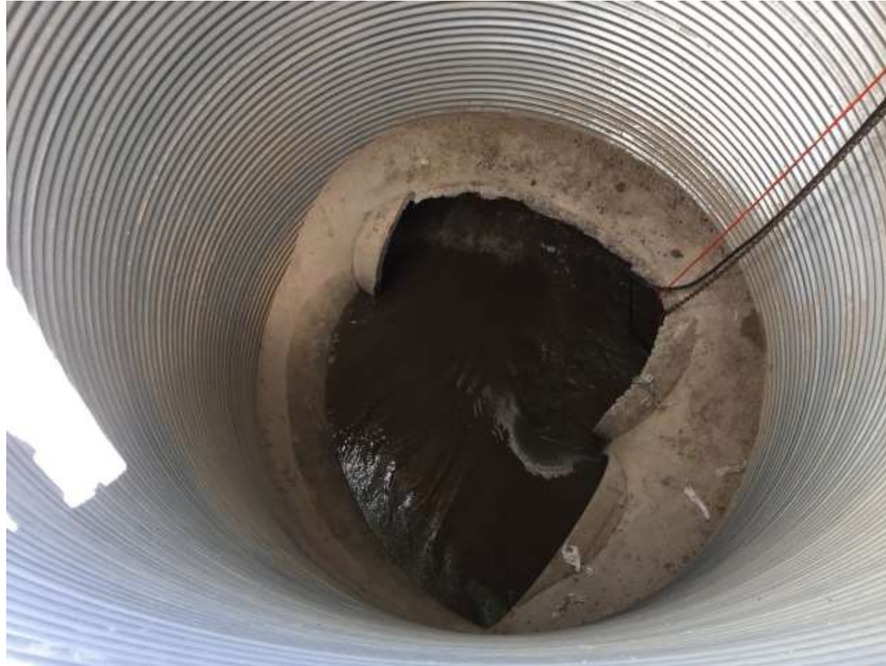
Downstream View of the Bypass Installed at Crossland Blvd.
