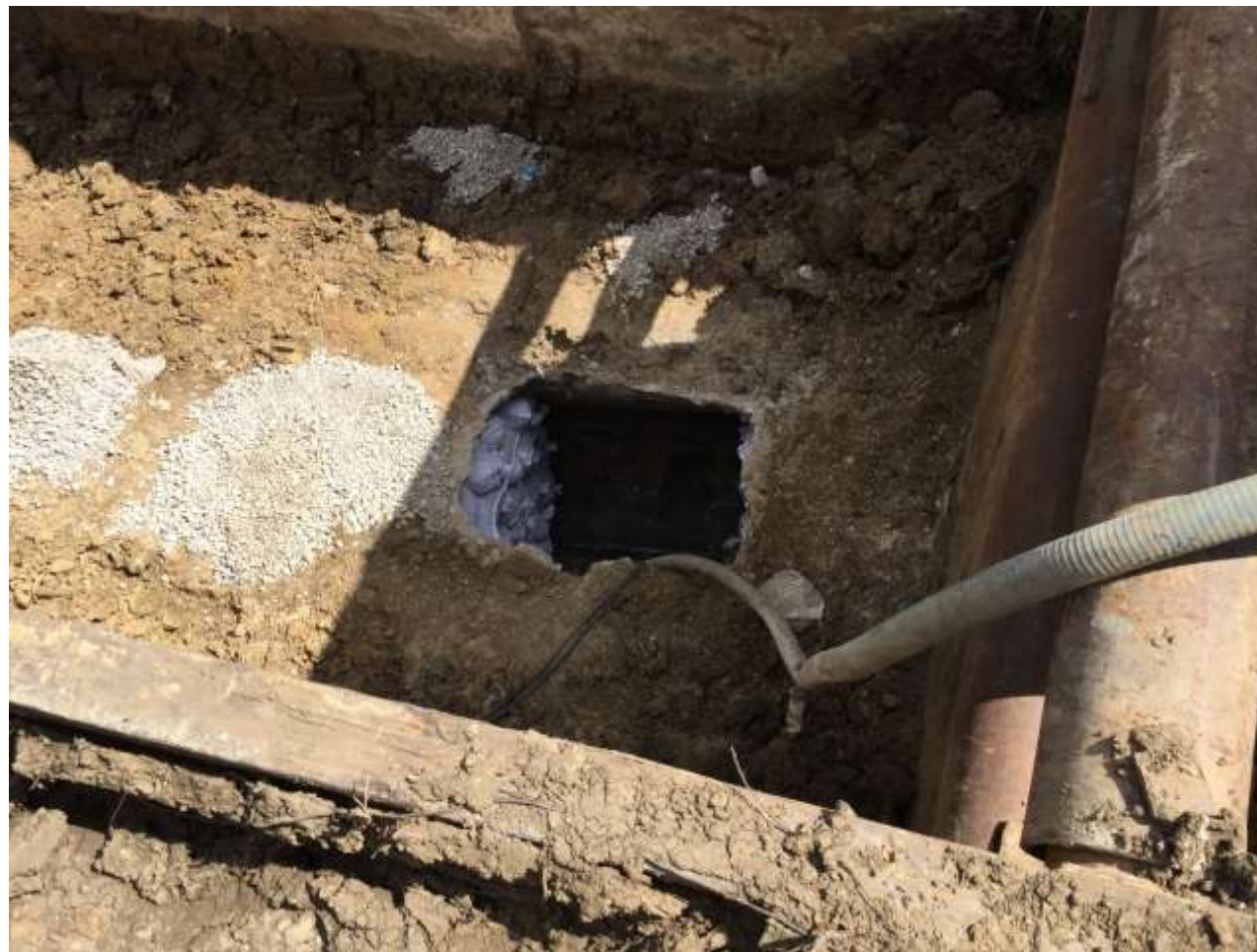
View of Plug Installed in Interceptor
