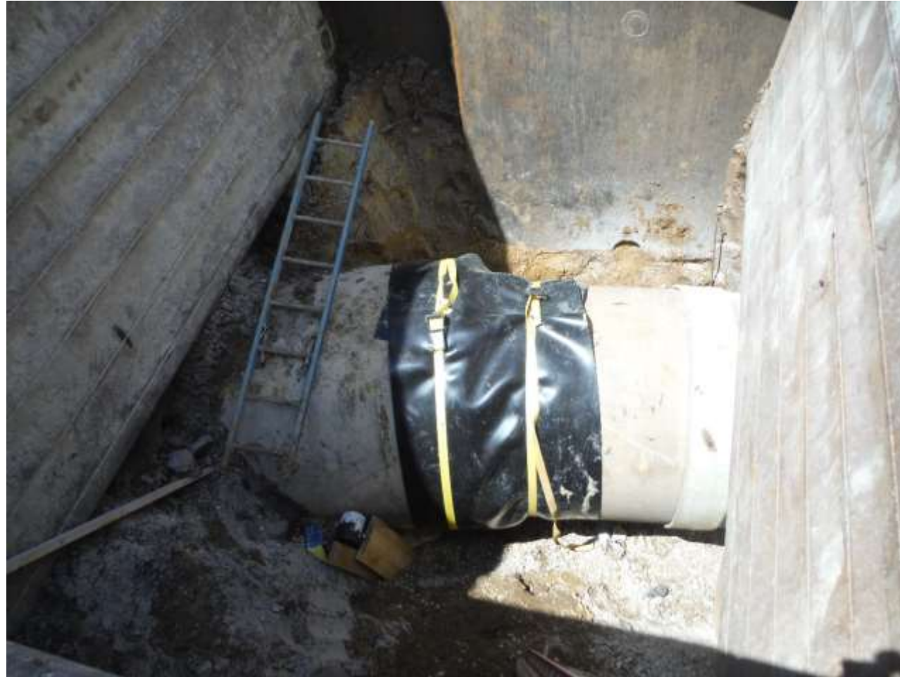
Connection to Existing 60" Interceptor
