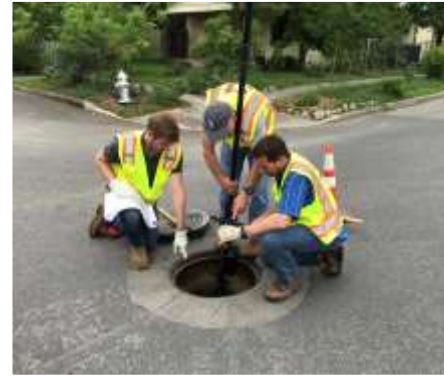
Manhole pole cameras
