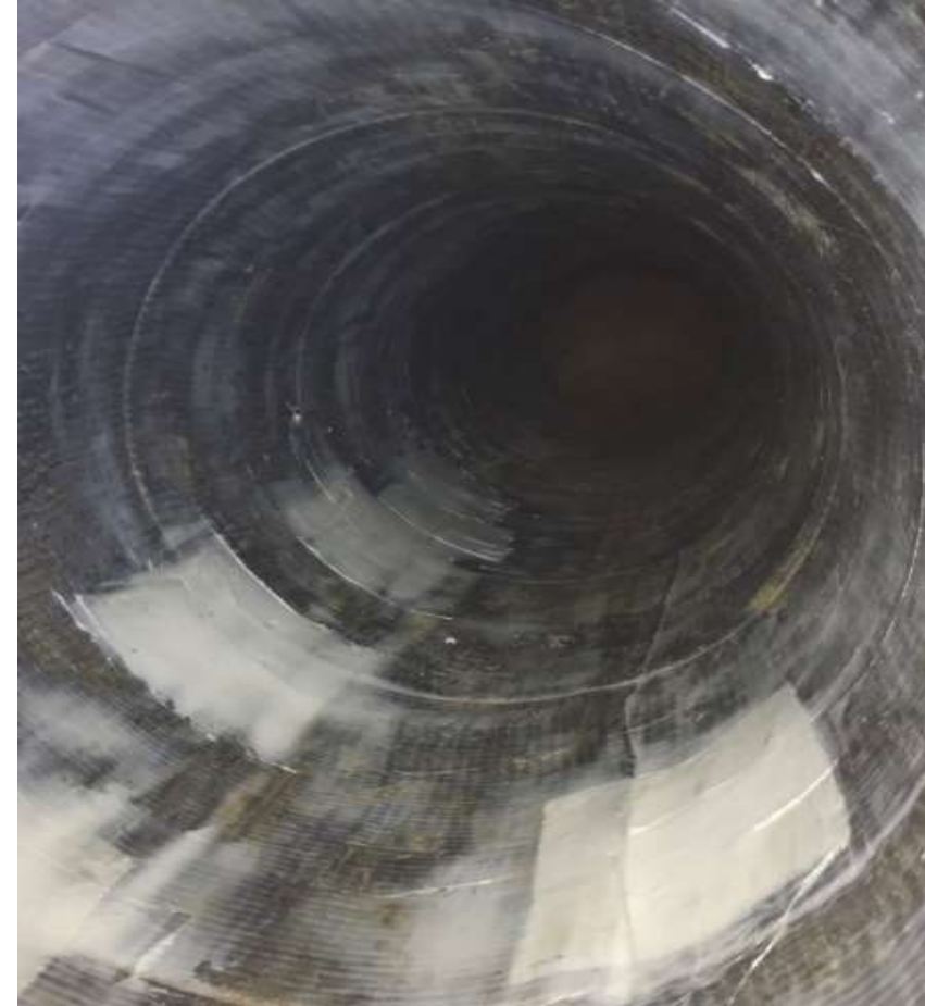
Completely Installed FRP System
