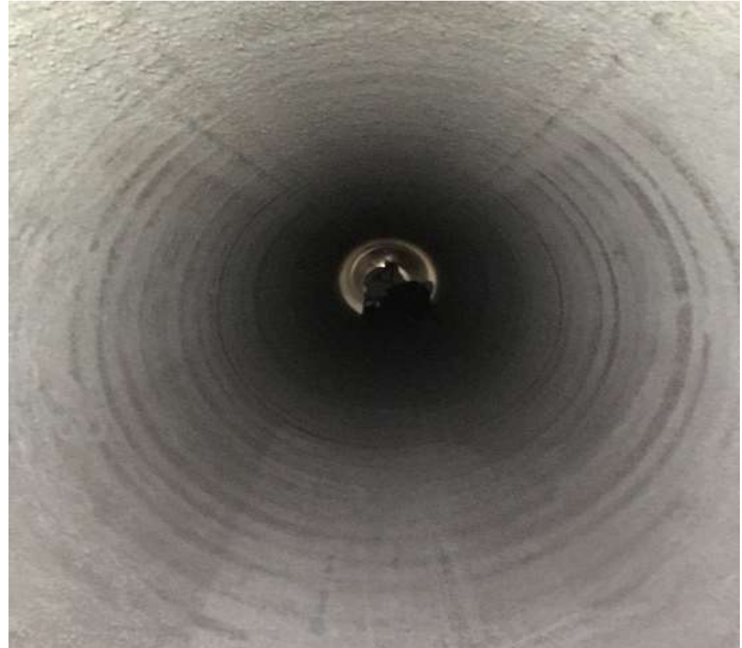
Finished Surface - Concrete
