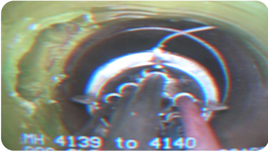
Post grouting mainline view of lateral connection.
