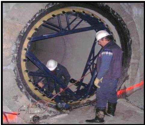
Mainline Test & Seal Packers available for 6" through 144" pipes.
