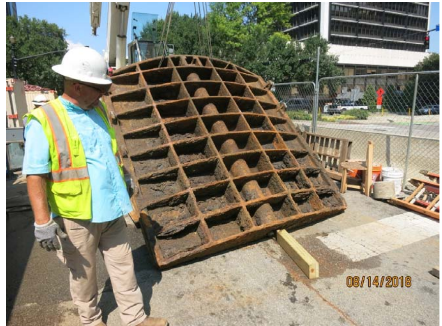
REMOVE & REPLACE SLUICE GATE
