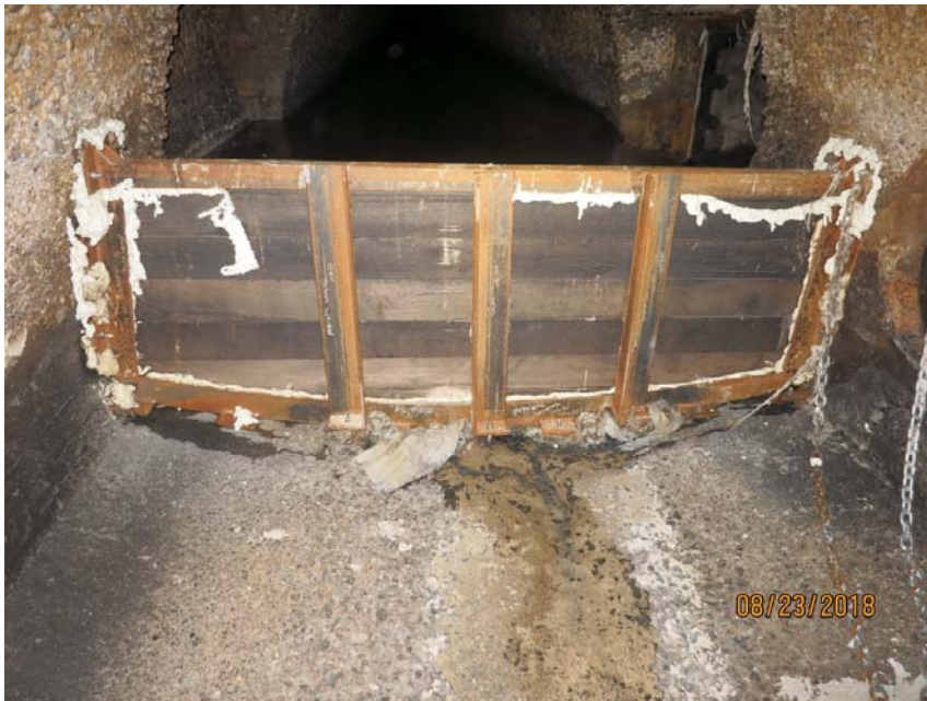
INSTALL PARTIAL HEIGHT WEIR
