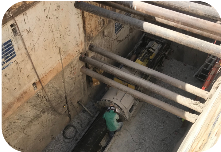
Engineered bore pits
