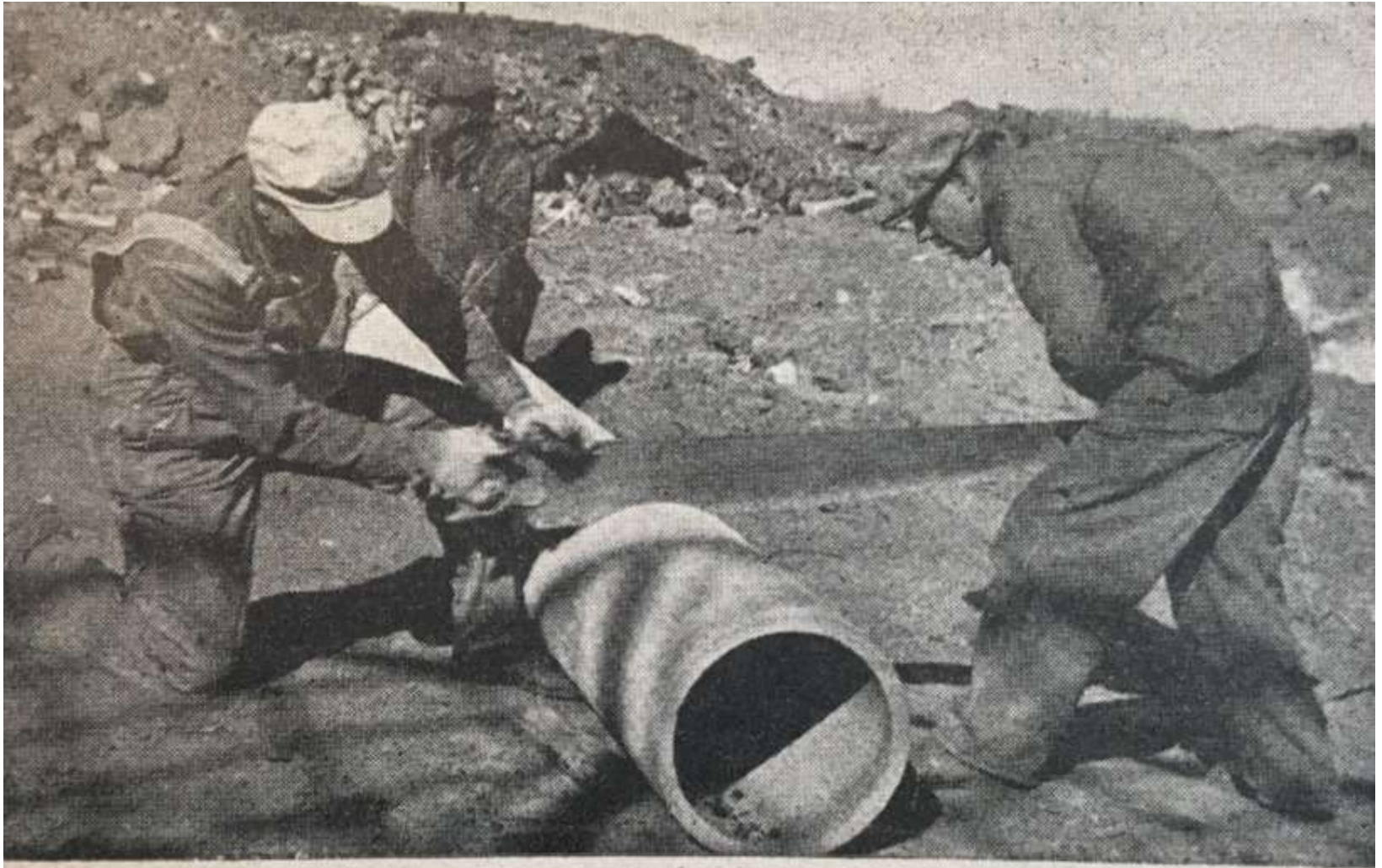
Cutting Transite Pipe with a handsaw
