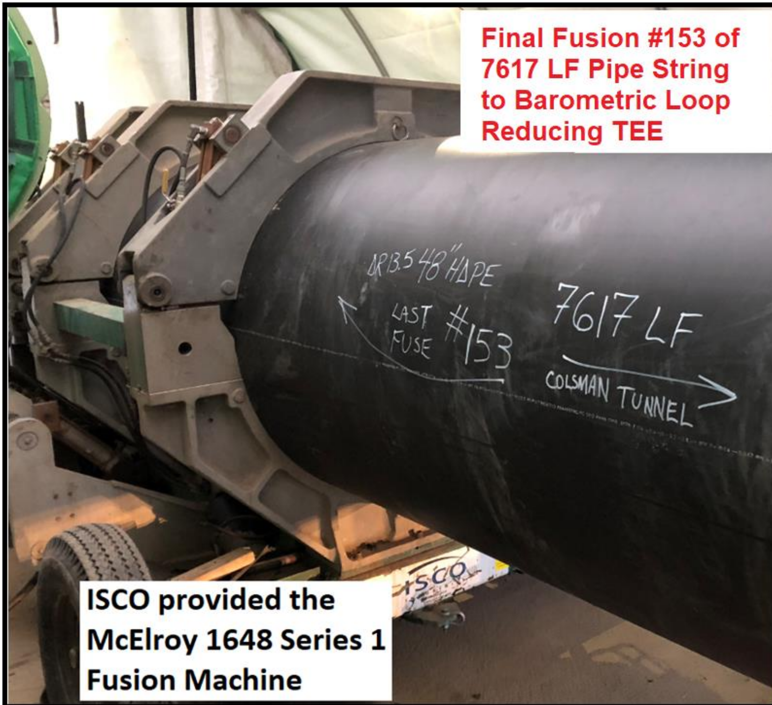
ISCO 48"x36"x24" Reducing Tee w/MJ adapters Fused at Max Rotation to enter Tunnel at Vertical
