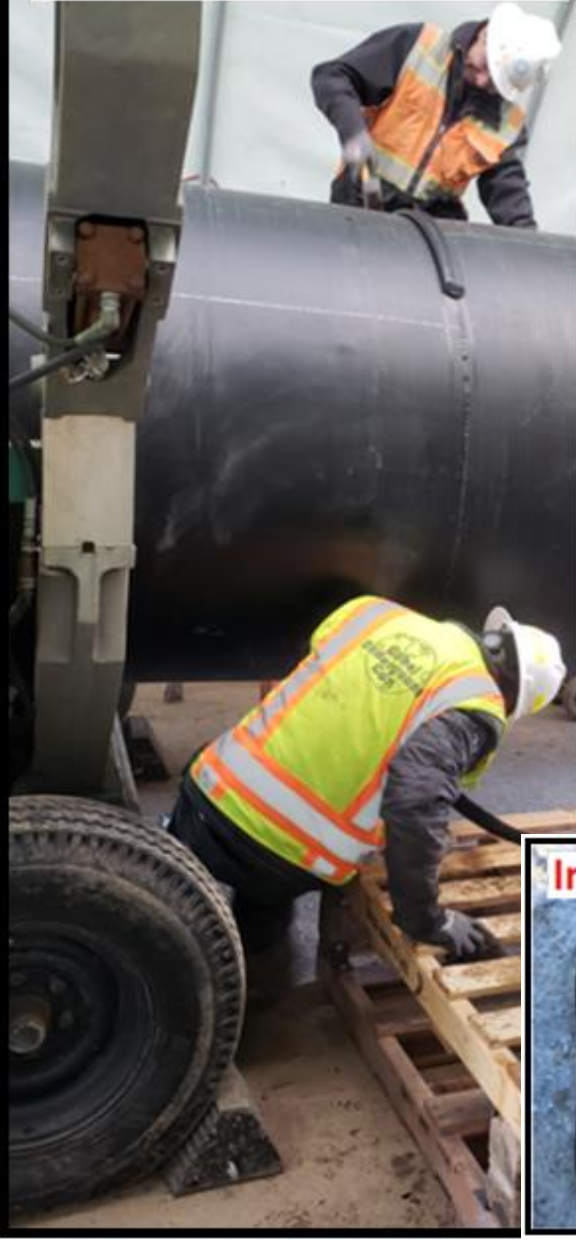
1922 LF of Exterior Bead removed by Hammer & Chisel
