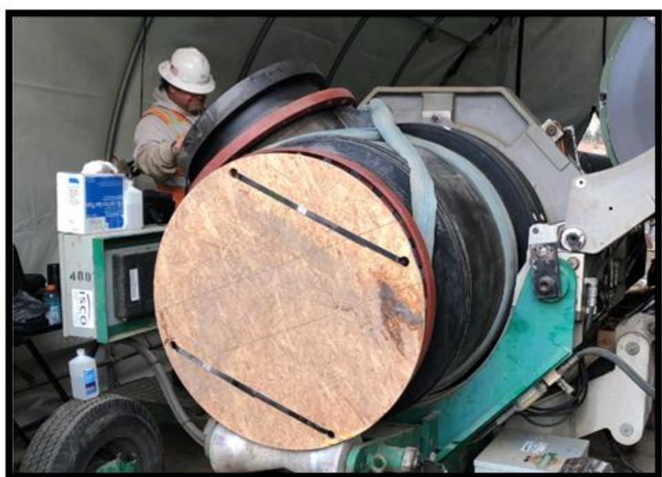
ISCO 48"x36"x24" Reducing Tee w/MJ adapters Fused at Max Rotation to enter Tunnel at Vertical
