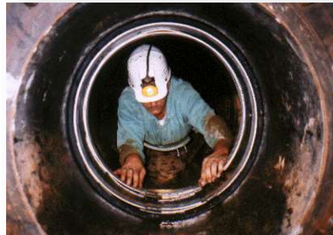
Install Retaining Bands
