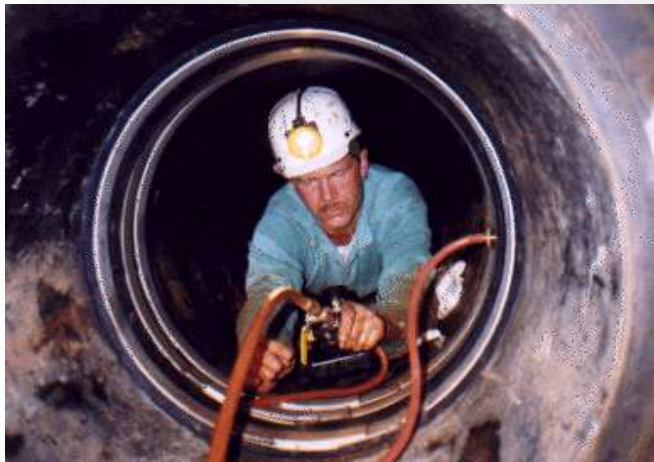
Pressure Test Seal
