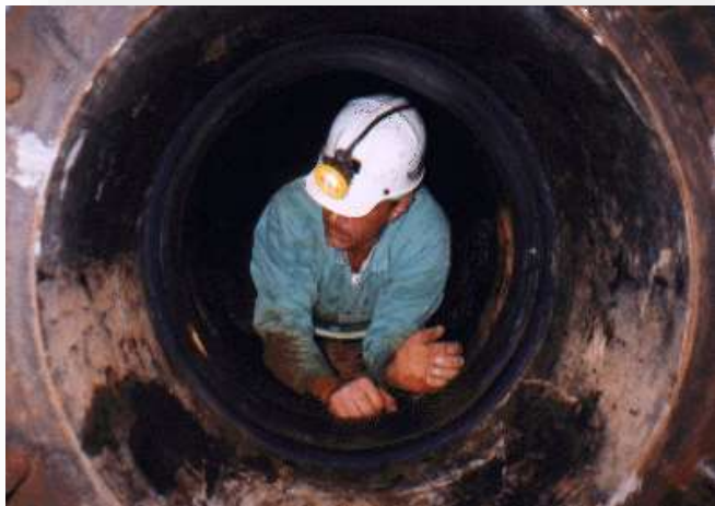
Install Rubber Seal
