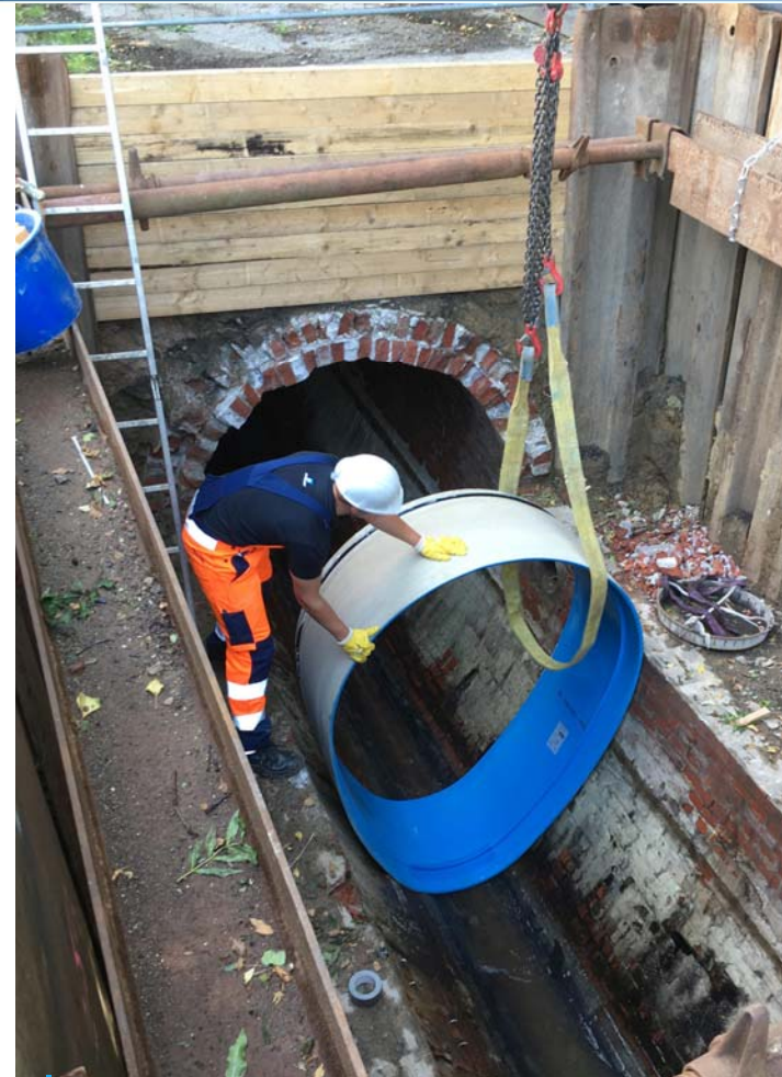
600 ft of 58" x 78" Egg Shape GRP in Germany.
