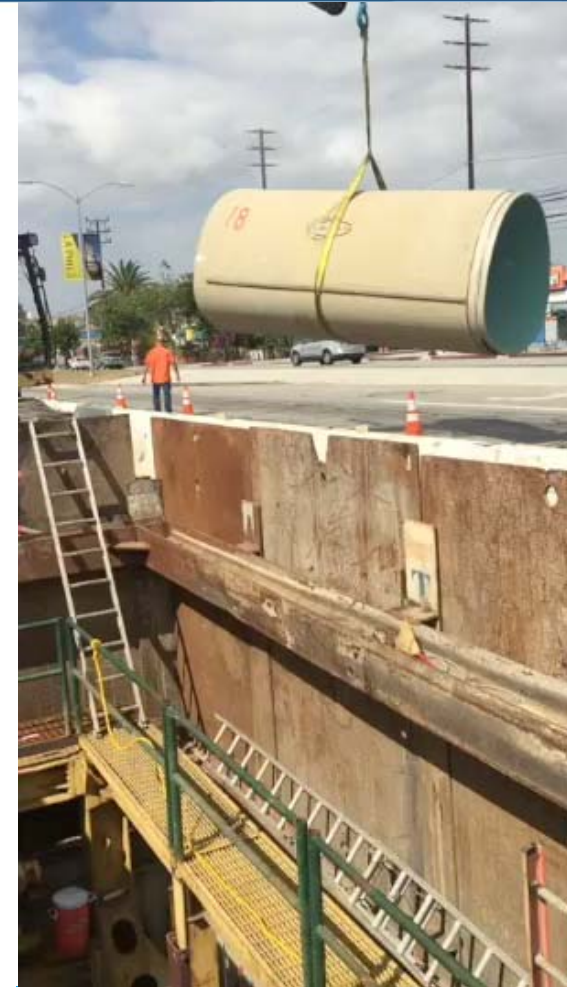
West Los Angeles Interceptor Sewer (WLAIS) Kelton to Overland 1650 LF of 58" x 52"
