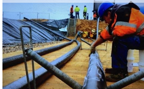
Cable pull-in lubrication
