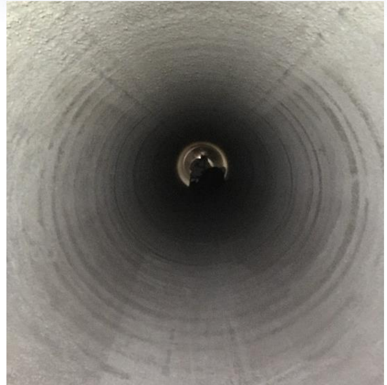
Finished Surface - Concrete
