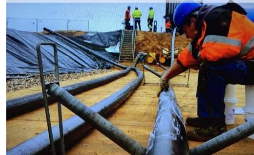
Cable pull-in lubrication
