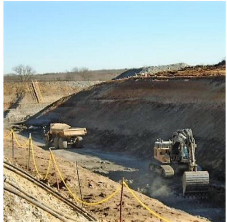
Excavating the Intake Tower Conduit January 2019
